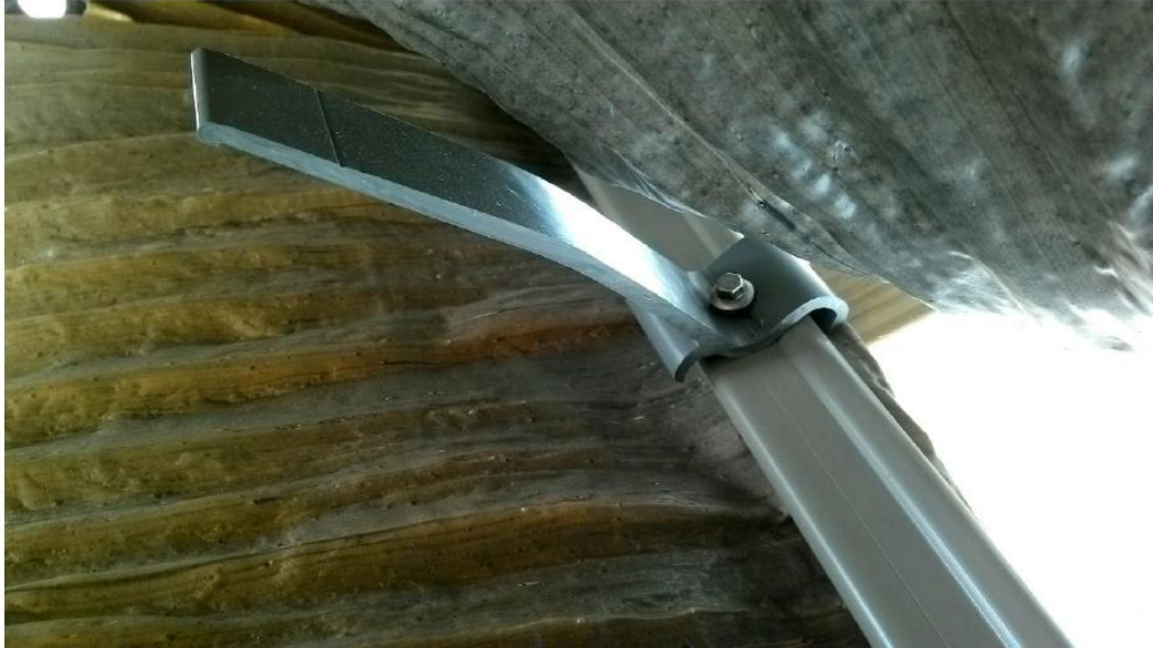
Representative Photograph Deck #2: One clip exhibits permanent deformation.
