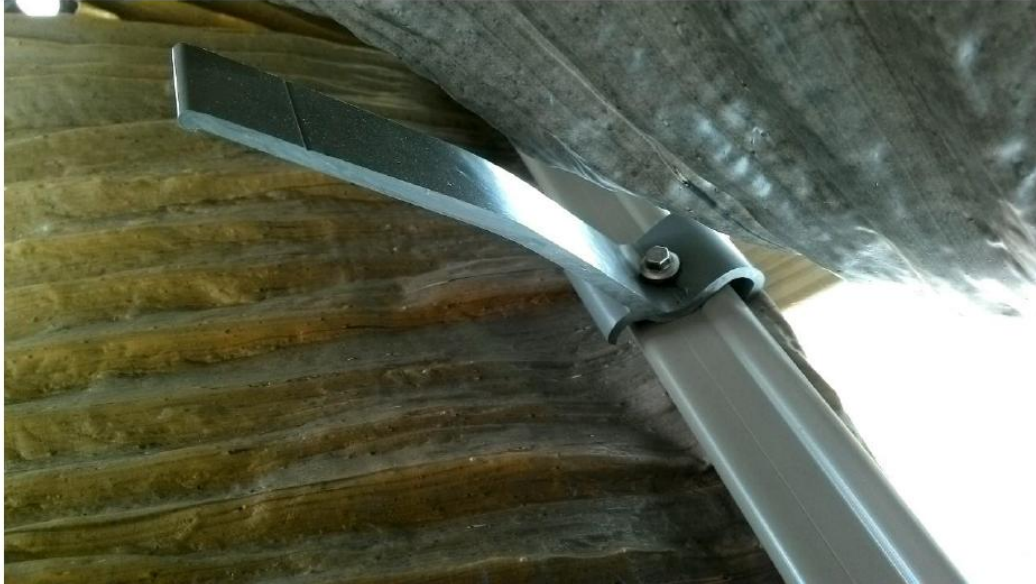
Representative Photograph Deck #2: One clip exhibits permanent deformation.
